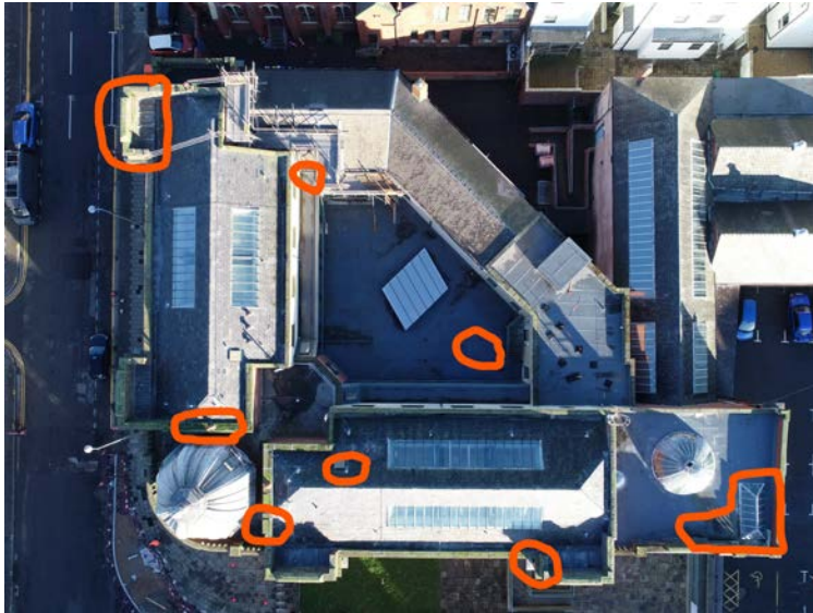
Central Roof leaks image - areas of know water egress and damp.
